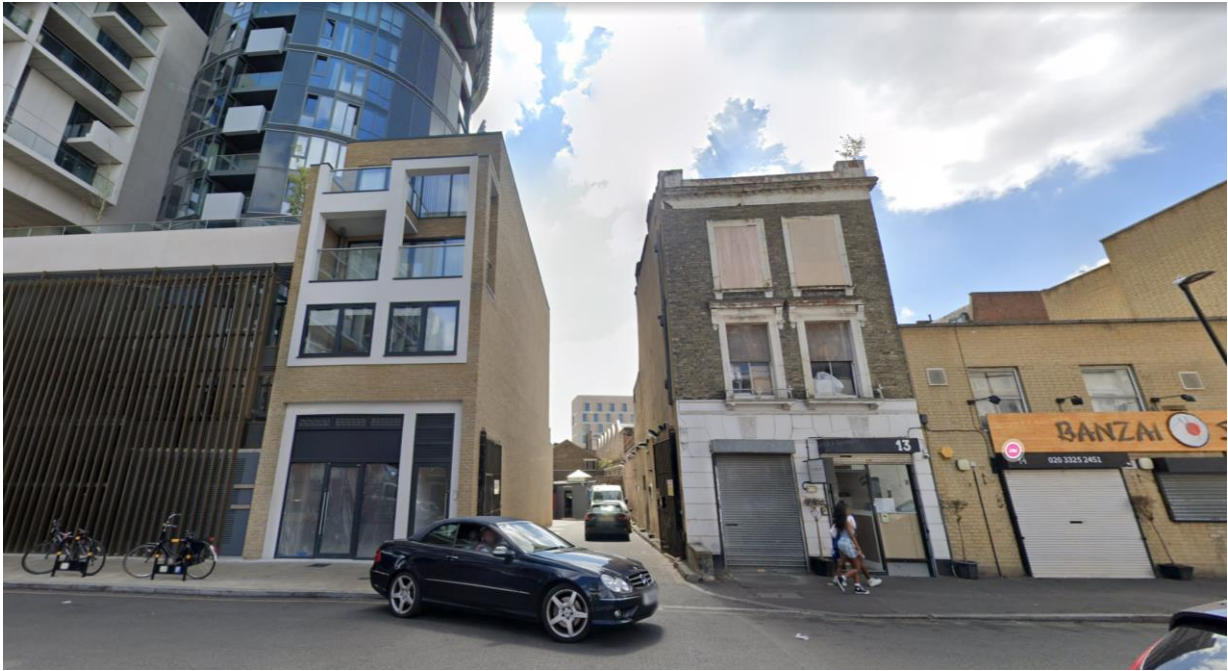
Fig 7: Front elevation of 13 Goodwin Street with service yard separating it from 11 Goodwin Street. This space is not within the site curtilage.
